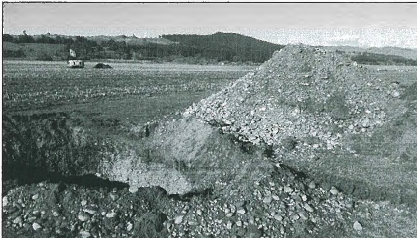
Photo showing material excavated from trial pit Test Pit D.
