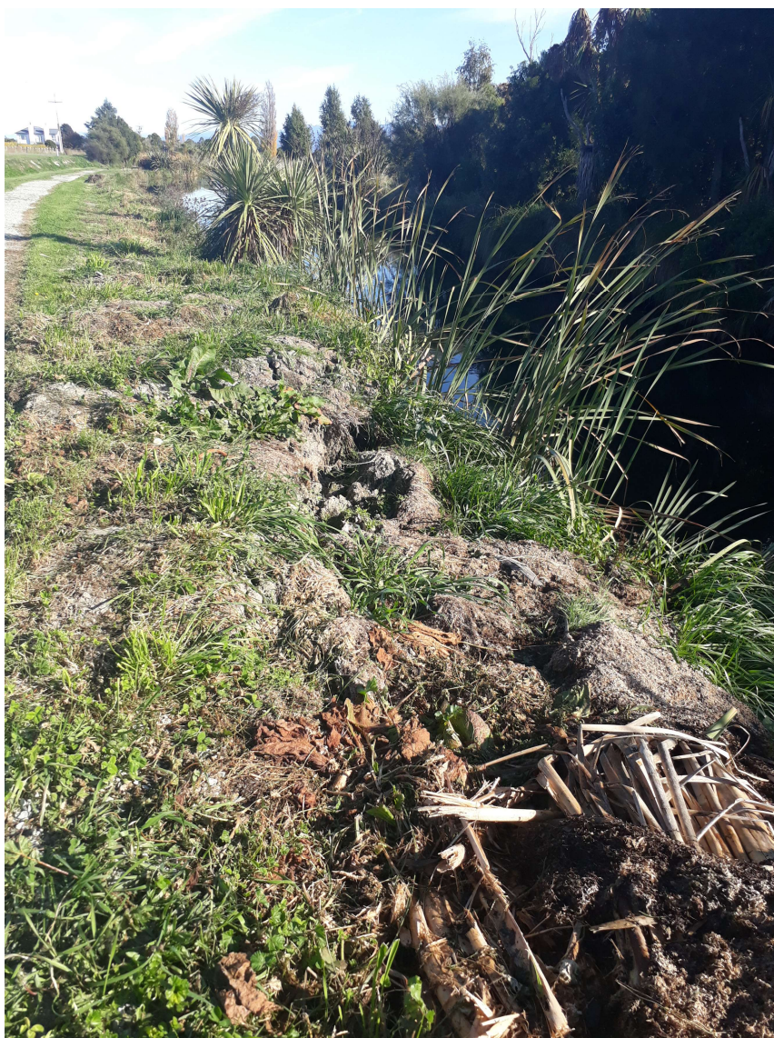
Figure 2 - Slumping of the Lagoon bank
