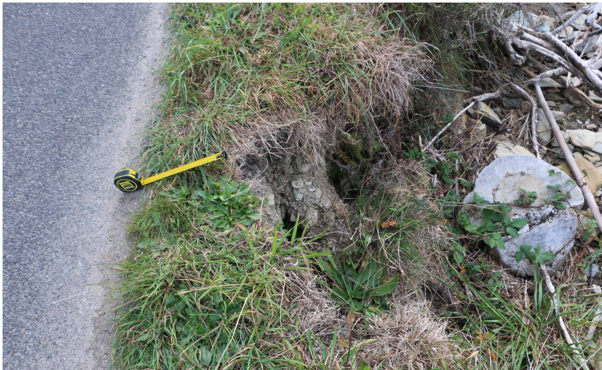
Photo: Narrow (300 mm) road shoulder due to tidal erosion on the Mahakipawa Causeway
