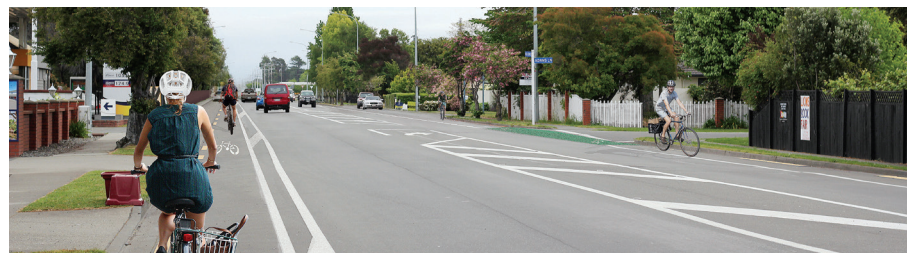
This image shows the proposed new configuration of Middle Renwick Road, looking west
